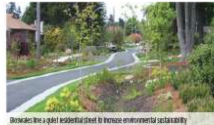
Bioswales line a quiet residential street to increase environmental sustainability
