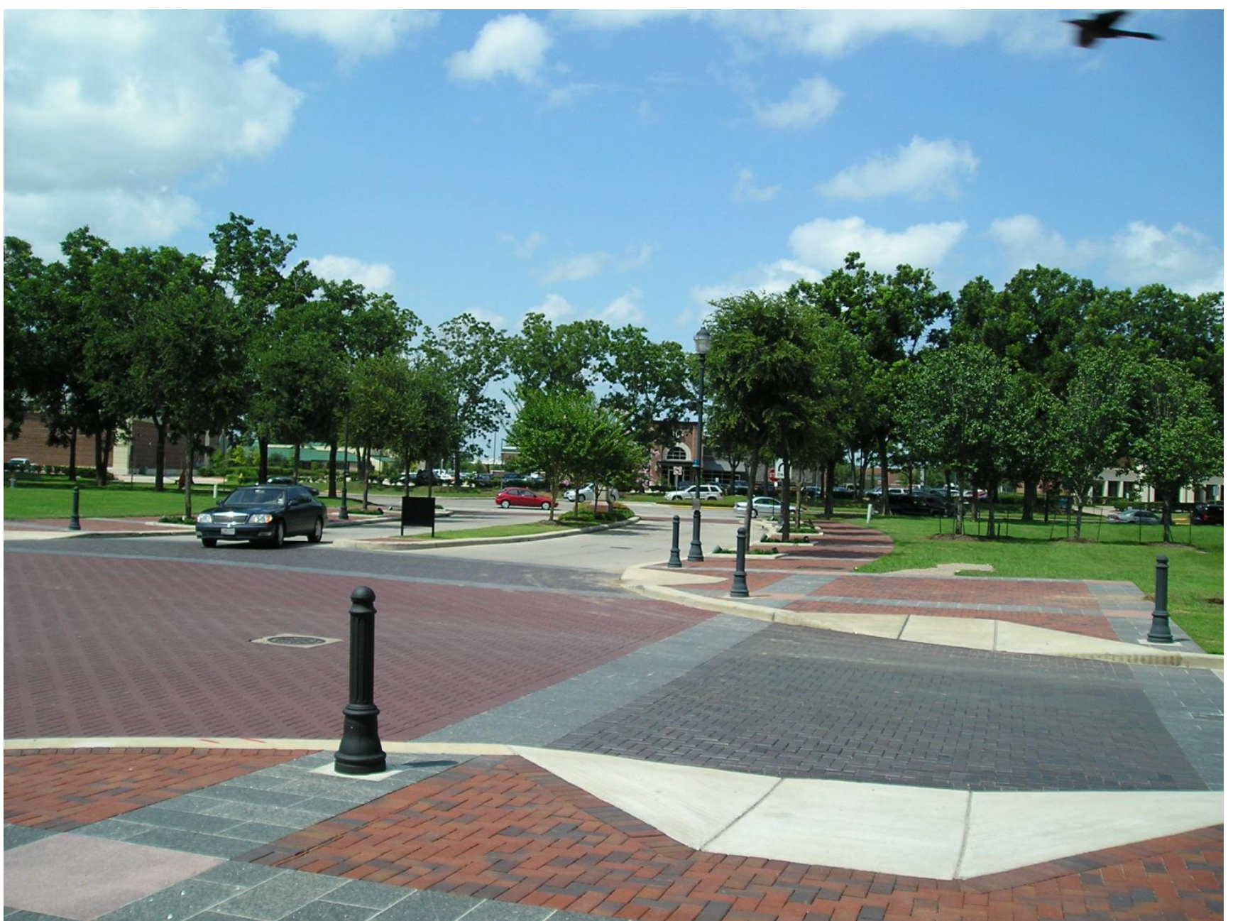
Sugarland, TX – Textured Intersection and Ped Crossings
