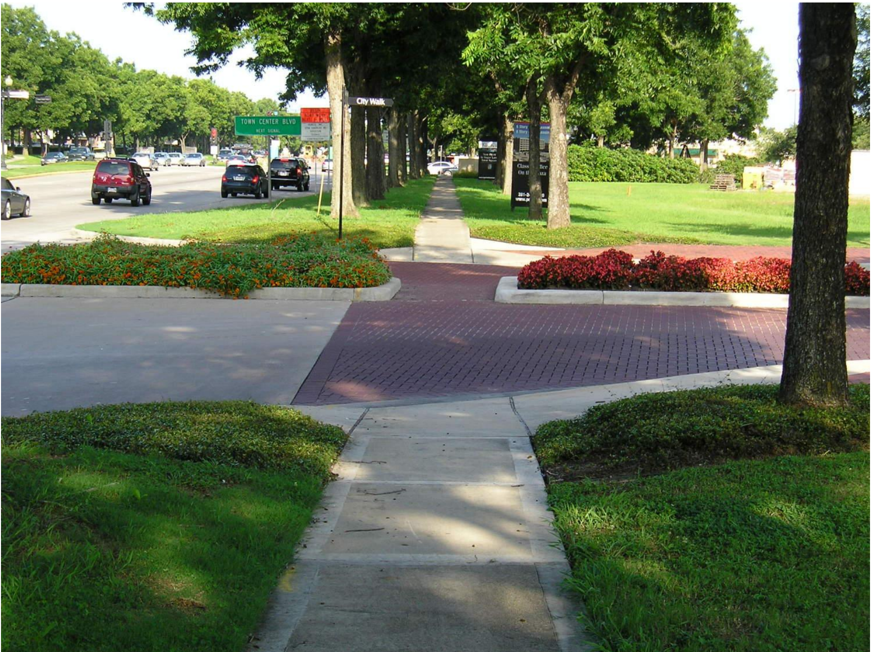
Sugarland, TX – Textured Ped Crossing with Planted Median
